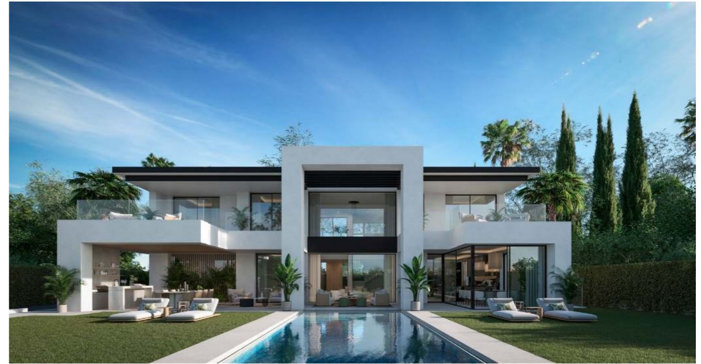
Façade of the garden area of the house.
